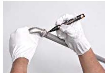
**Marking the insertion depth:** The tube must be fully inserted into the fitting until it reaches the tube stop in order to make a perfect joint. Marking insertion depth will ensure that any tube movement is detected, which is especially important if the joints are to be pressed at a later time.
