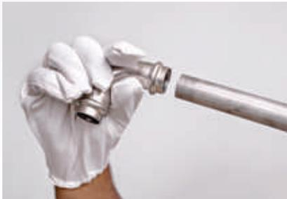
**Assemble fitting on tube:** To assemble the joint, the tube must be inserted into the fitting up to the tube stop. (Use the mark on the tube which was made earlier as reference). The pressing operation should only be undertaken when the tube reaches the tube stop.
